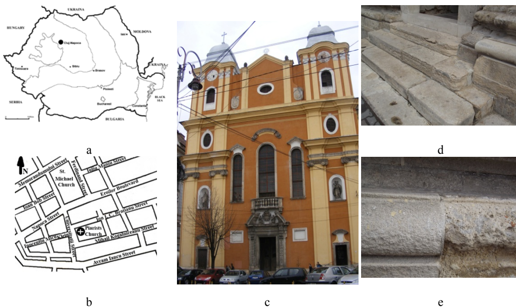
Fig. 1 – The Piarists Church from Cluj Napoca: localization of Cluj-Napoca area on Romania map (a); the Piarists Church on the map of the Cluj-Napoca centre (b); North-west facade of the Piarists Church (c); eroded steps in the north-west facade of the building (d); different erosion of limestone from the same cornice at the north facade (e).
